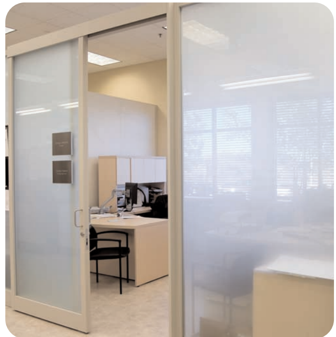
TIMES CHANGE Much of the space features moveable walls which can easily be moved and reconfigured as the need for available space changes over time.
